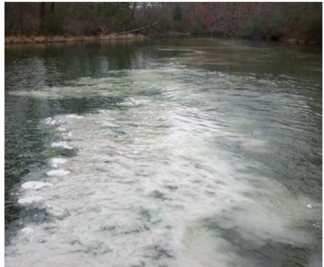
Figure 7. Lime is washed from a barge using a high-pressure hose and is thoroughly mixed throughout the pond.
