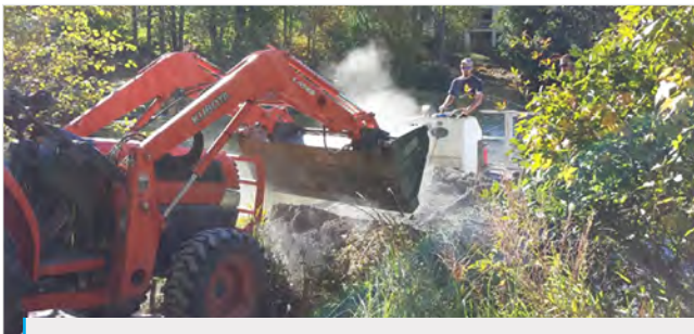
Figure 6. Crushed lime is loaded onto a barge to be applied to larger ponds. Since lime application may be more than a ton per acre and require the application of large quantities of material, many landowners choose to hire one of the numerous pond and lake management companies in Texas to apply lime to their ponds.
