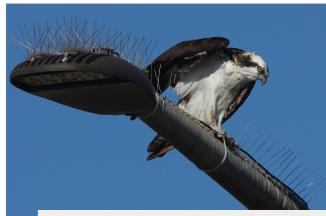
Figure 7. Bird spike perch deterrents should be resistant to bending so that larger birds cannot manipulate them into a perch. Photo by R.J. Adams
