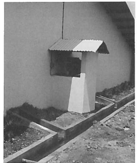
Photo 11. Air blower for Unit I Hatchery (high volume low pressure), later moved inside.
