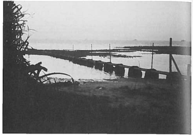
Photo 14. Concrete holds Intake Pipes in place, visible at low tide.
