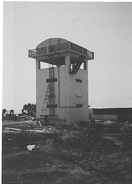
Photo 20. Elevated reservoir (50 MT) acts as a constant head device for Unit I and Unit II (U.V. treatment takes place in head device reservoir and pumps, and D.E. filters are housed in structure below elevated reservoir).
