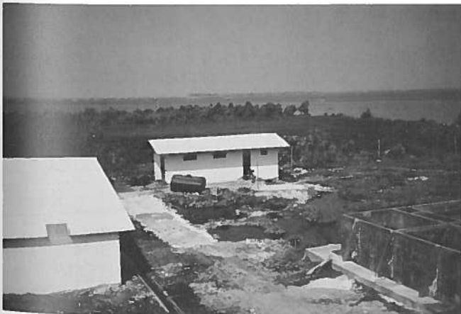
Photo 10. Maturation room (Unit II), lower left, generation or building, center; seawater settling, lower right.
