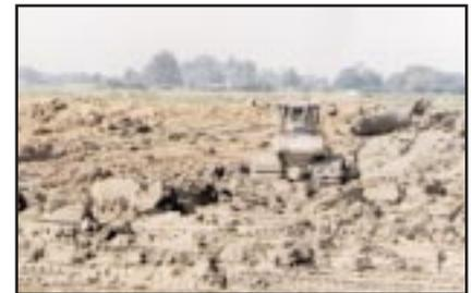
Figure 6. After material in the rows has dried to a heavy plastic consistency, pack the soil back against the levees.
