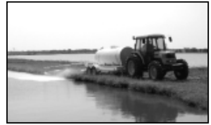
Figure 6. Hydrated lime slurry being applied with a pull-behind sprayer.
