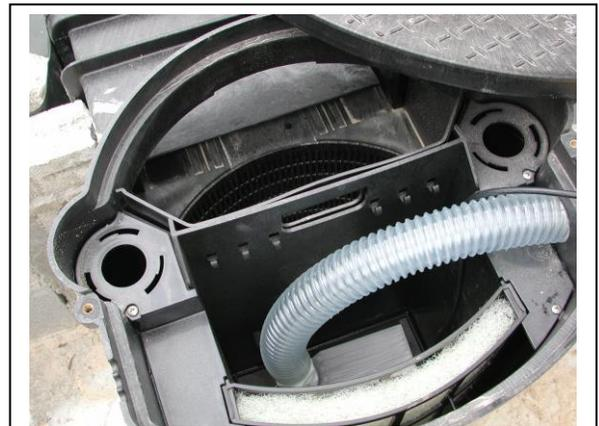
This mechanical filter collects leaves and larger debris in the reservoir while the fiber and foam filters help trap particles of dirt and organic matter.
